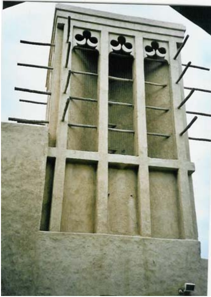
Building Construction. Fig. 17 Wind catcher tower (Dubai) (photo by the author).
